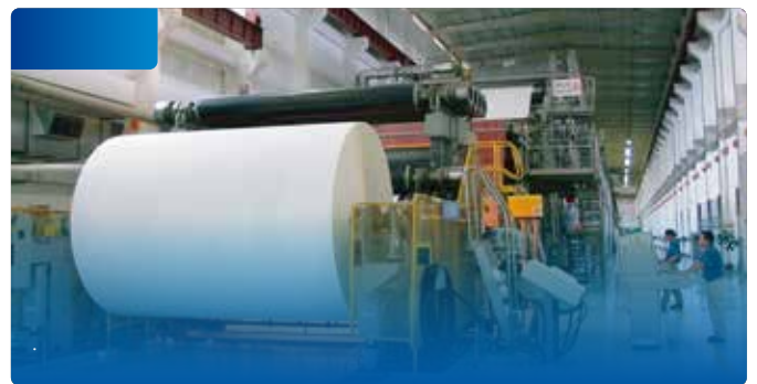
Papermaking: pulper, grinder, pulveriser, papermaking machine, rewinder, etc.
